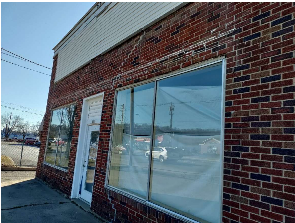
Figure 4: Stairstep cracking repairs on the east wall of the building to the south of the addition site.
