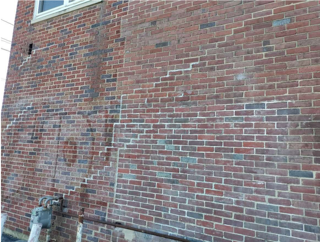
Figure 5: Stairstep cracking repairs on the north wall of the building to the south of the addition site.
