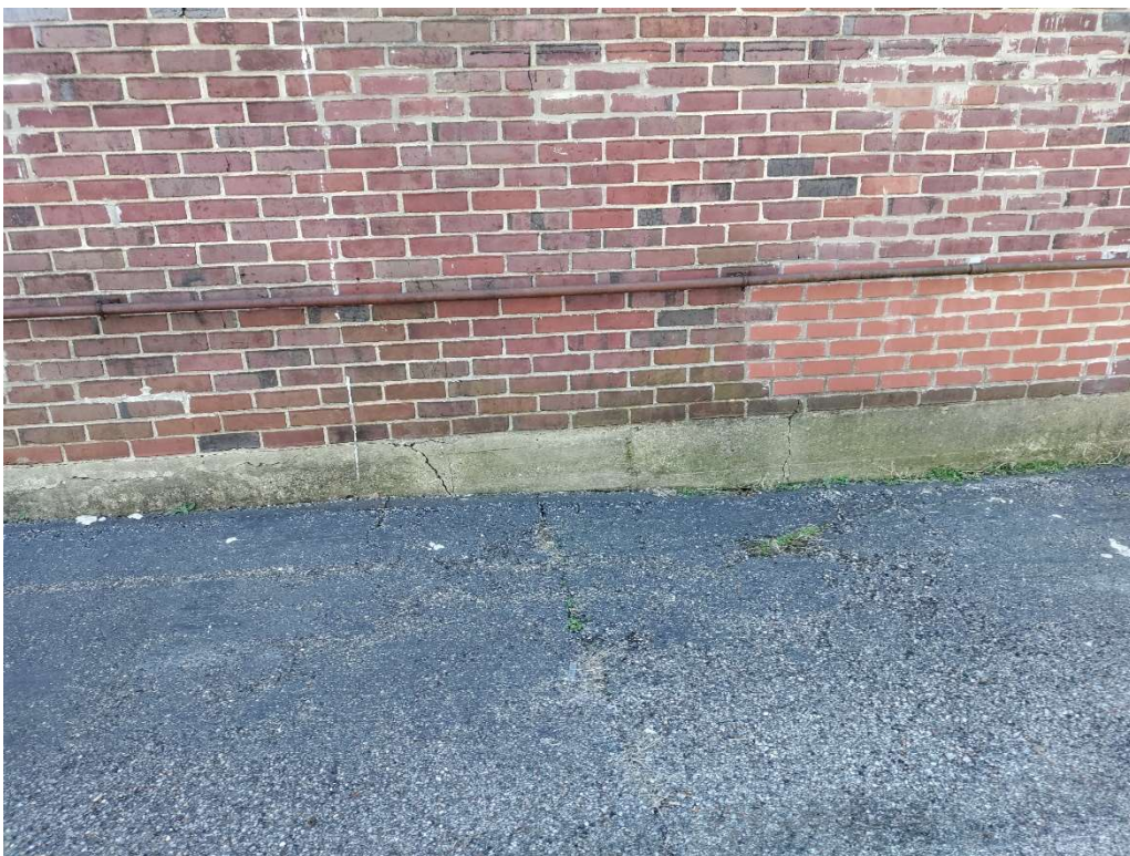
Figure 6: Cracks in the footing wall of the building to the south of the addition site.
