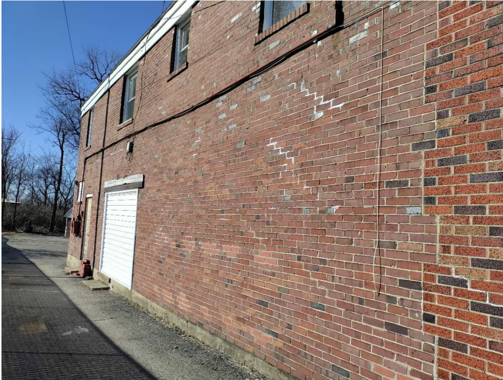
Figure 3: Stairstep cracking repairs on the south wall of the building to the south of the addition site. This type of cracking is commonly observed in buildings experiencing differential settlement.
