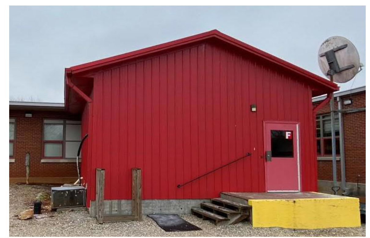
7 Existing Photo - F NTS
