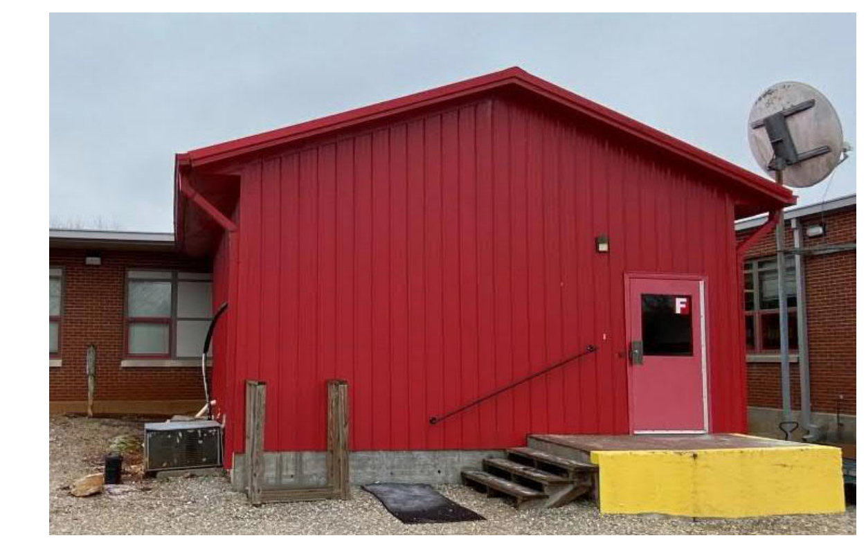
7 Existing Photo - F NTS
