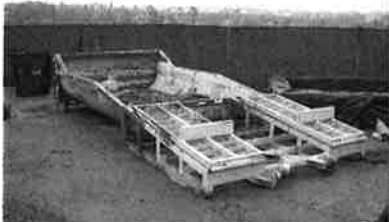
This is a commercial concrete washout tank with fold-up ramp.
