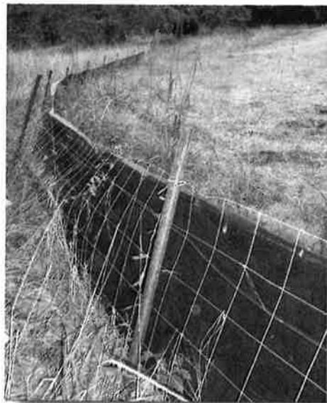
Good installation of "super" (i.e., wire reinforced) silt fence. Note that wire is installed between the fabric and stakes, and provides a web of support as the ponded flow pushes against the fabric. Also, note the grass strip between the bare area and the fence, which helps to slow and filter flows before ponding along the fence line.
