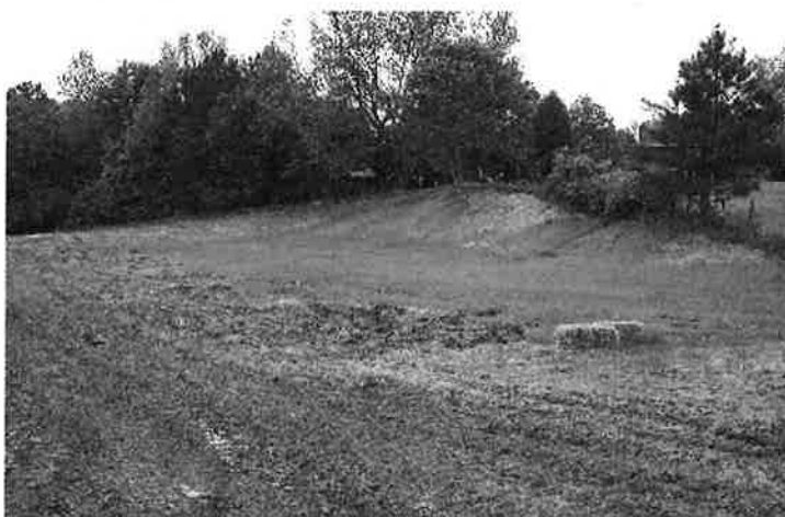
Designate haul roads and material storage areas on large sites, and seed or mulch the rest to minimize the amount of bare areas exposed to the weather. KPDES regulations require that portions of the site that have not been worked for 14 consecutive days be temporarily or permanently stabilized with seed and/or mulch.
